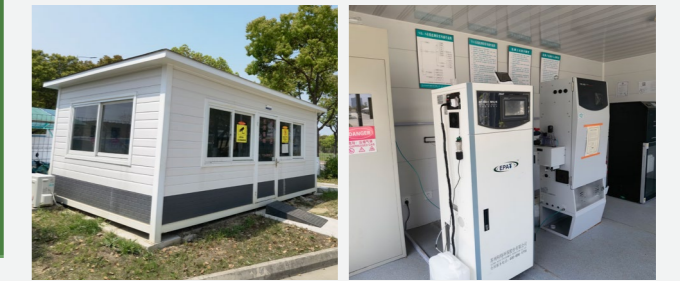
automatic monitoring station and automatic monitoring facilities at Hengrui Pharma sewage discharge outlet
